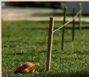
1. Stake out the fence line.
