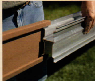
5. Slide bottom rail over the metal insert.*
