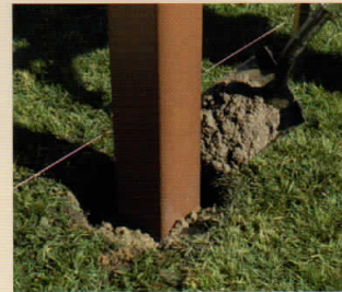
3. Set posts in concrete.
