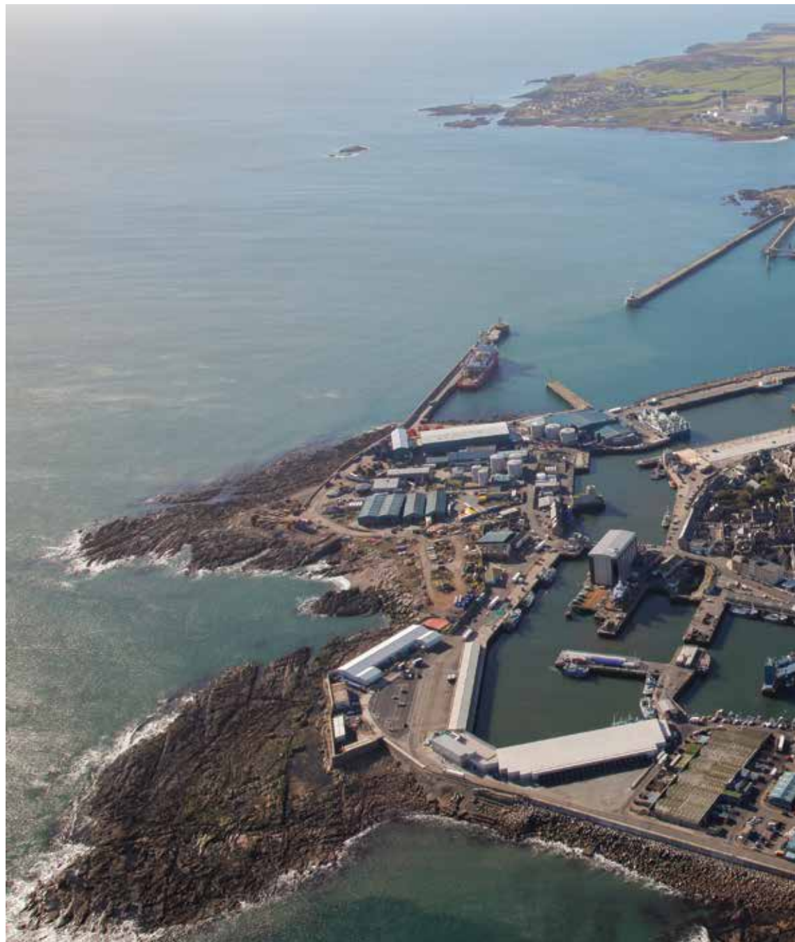
Aerial view of Port of Peterhead. Photo: Port of Peterhead.
