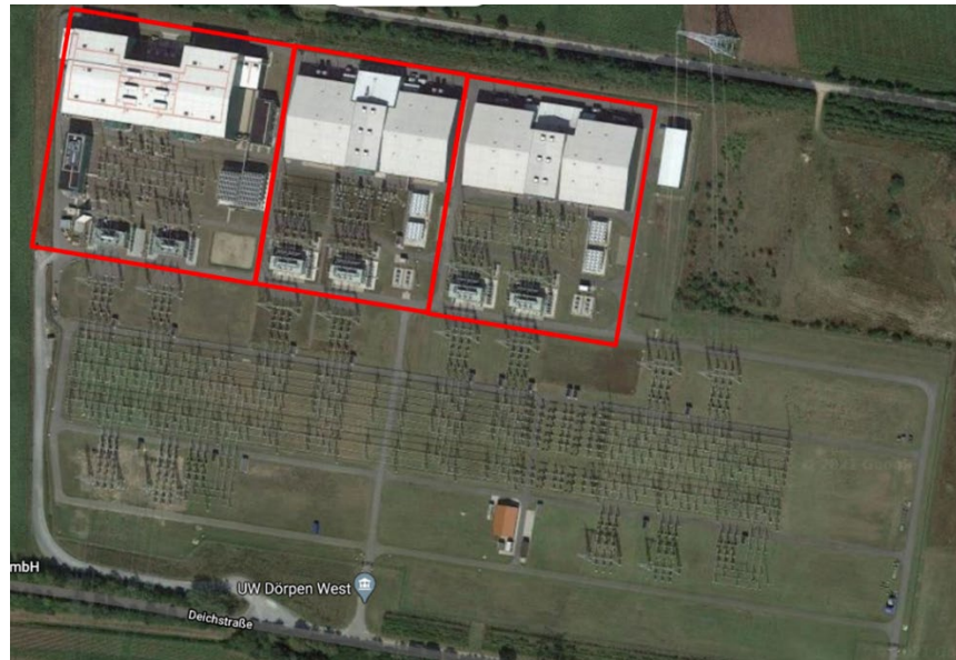
FIGURE 51. AC GRID VONNECTION OF THREE HVDC CONVERTERS FROM TWO DIFFERENT VENDORS
