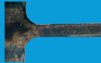
Minimal corrosion. The grid is completely intact.
