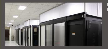
Floor Mounted Hot Aisle Containment
