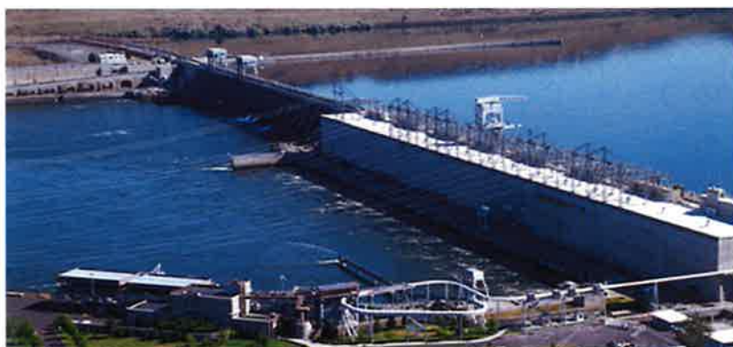
Federal Columbia River Power System (FCRPS)
