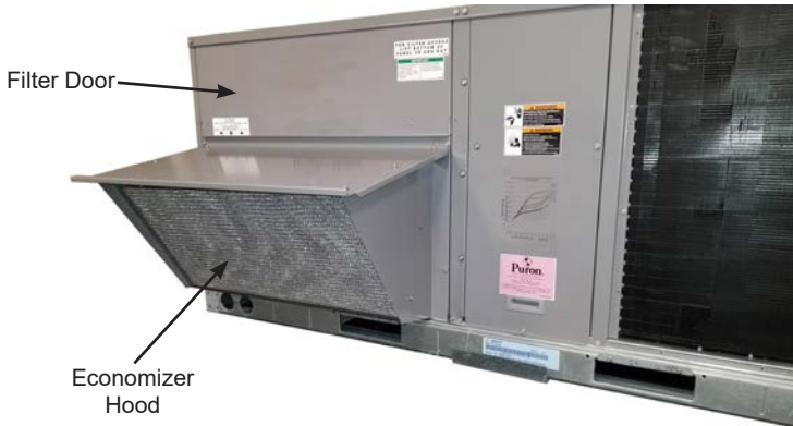
Figure 20 – Install Economizer Hood and Unit Filter Access Door
