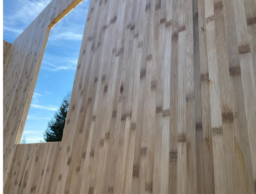
Figure 1. House Under Construction Using BamCore® Panelized Prime Wall™ System
