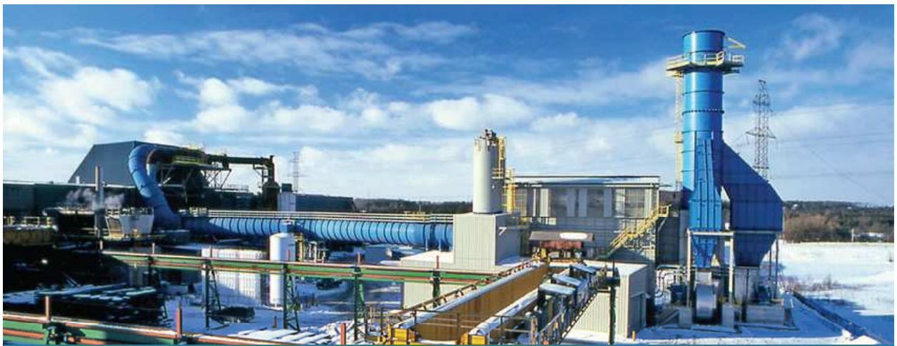
Gerdau's steel mill in Cambridge (Canada)
