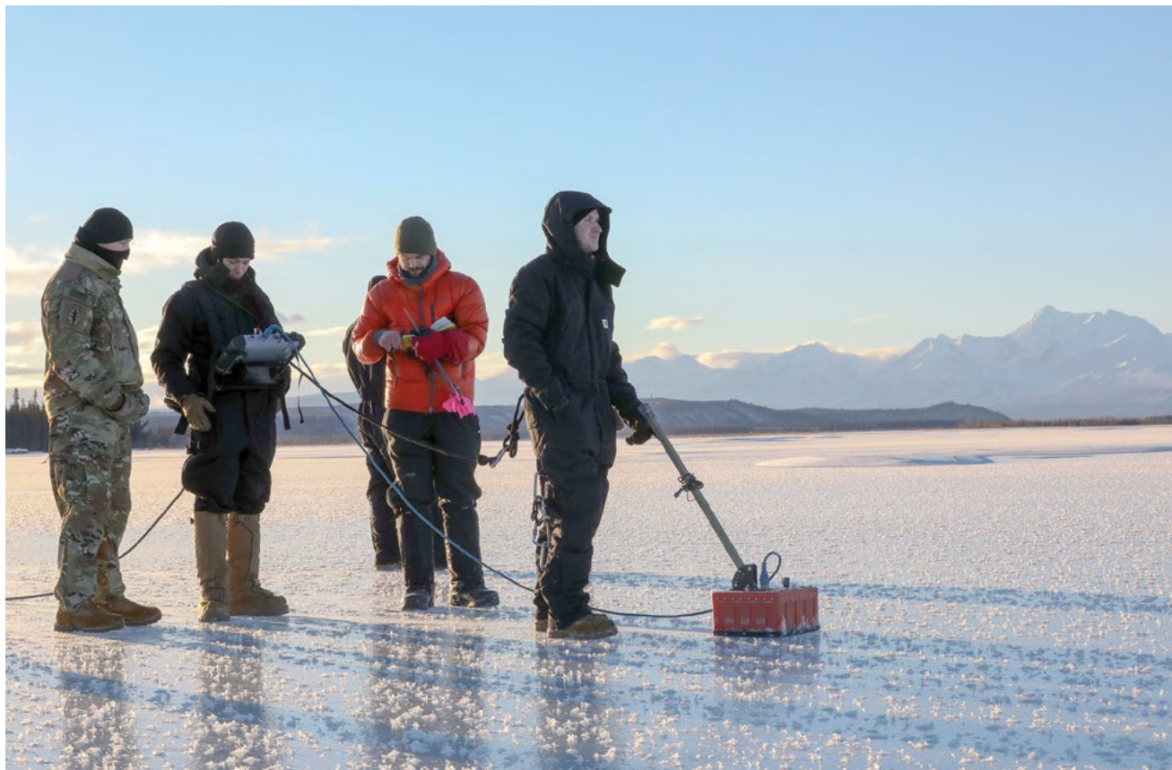
Paratroopers with 6th Brigade Engineer Battalion, 4th Infantry Brigade Combat Team (Airborne) (BTC[A]), 25th Infantry Division (ID), use ground penetrating radar to check the thickness of ice as they prepare to construct a bridge across the Tanana River at Donnelly Training Area, Alaska, 20 January 2021, in preparation for exercise Arctic Warrior 21. On 6 June 2022, the 4th Infantry BCT(A), 25th ID, was reflagged as 2nd BCT under the reactivated 11th Airborne Division as part of the U.S. Army's new arctic strategy. (Photo by Staff Sgt. Alex Skripnichuk, U.S. Army)
