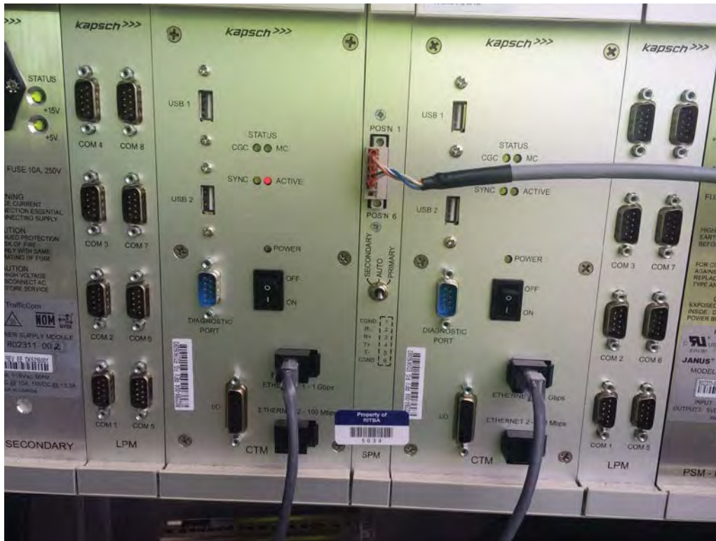
Exhibit 8.1-1: AVI Reader, RF Module, and Antenna
