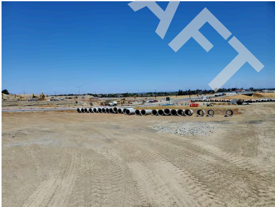
4 - Concrete piping stored on Site.
