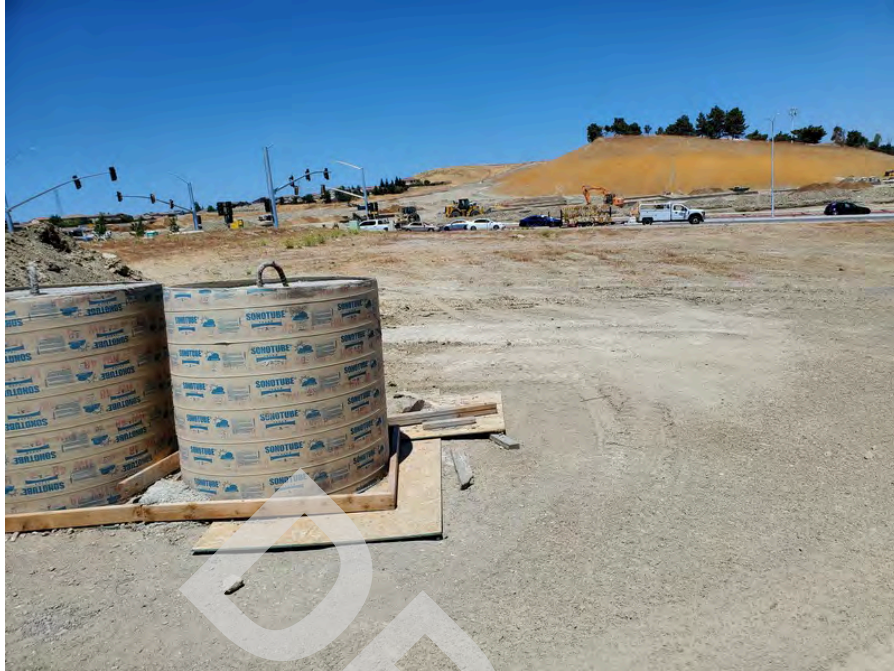
3 - Construction materials stored on Site.
