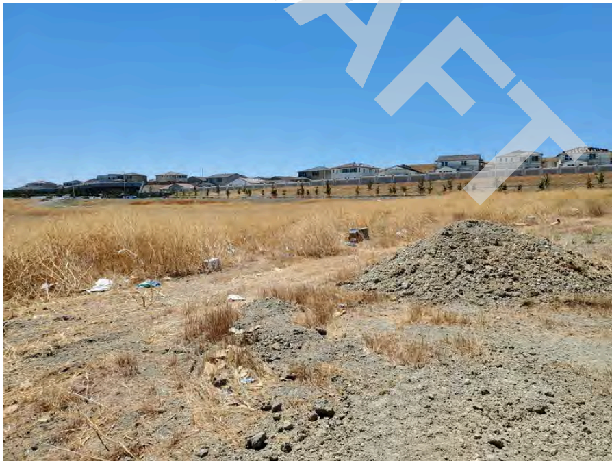
16 - Refuse and debris located in the center of the Site.
