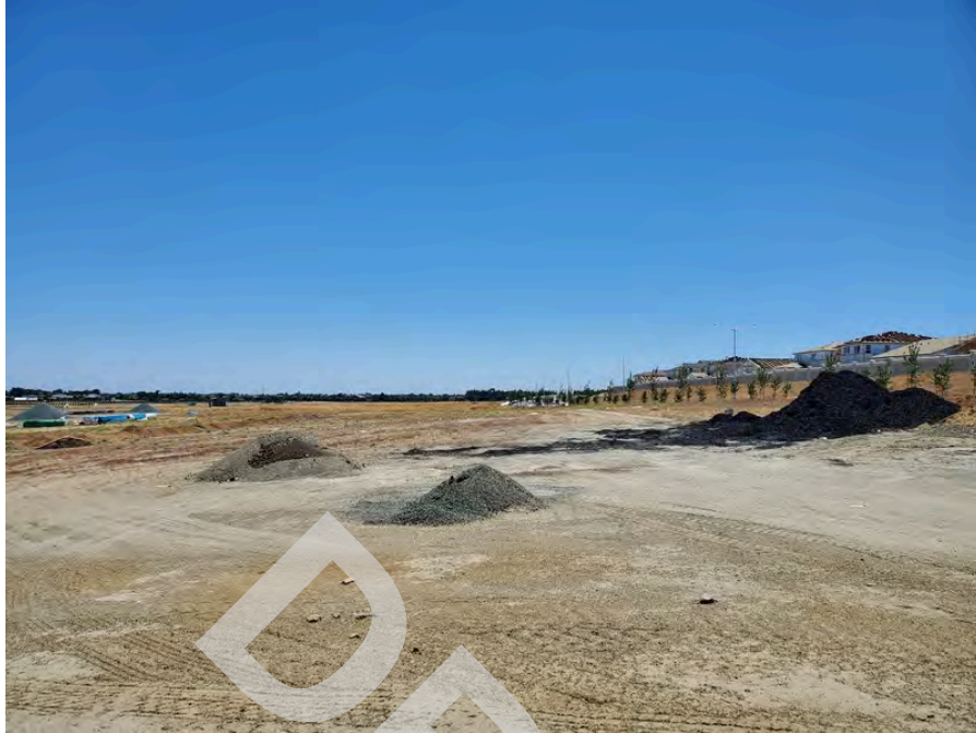
5 - View of the site from the northwest looking southeast.
