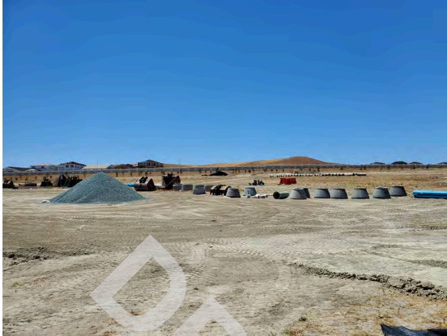
11 - Construction materials located in the central portion of the Site.
