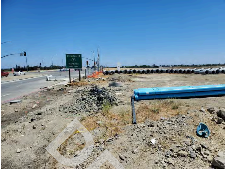
7 - Construction materials located at the northern corner of the Site.
