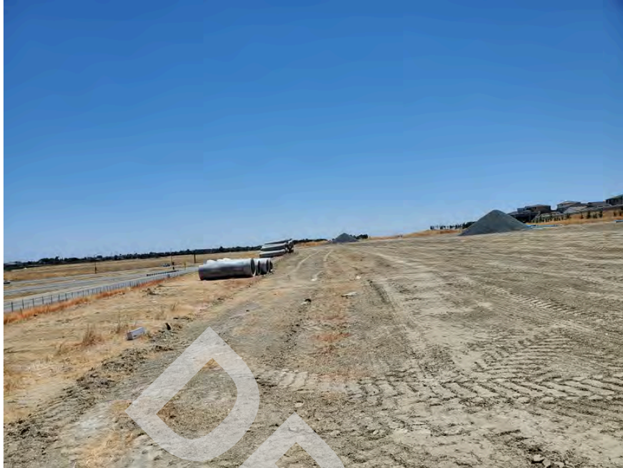
15 - View looking southeast from the northeast.
