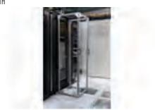
The Air Booth is a three-sided containment system that is placed directly over a perforated tile, in front of a rack or cabinet. This isolates the cold air provided from the perforated tile, creating a dedicated supply targeted specifically for the intake of active equipment within individual racks or cabinets.
