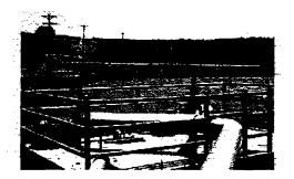
Shown here is a retention basin for capturing irrigation runoff and equipment for pumping captured water to a storage pond at a higher point in the nursery. There, the water can be mixed with fresh water and held for later use.
