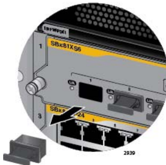
Figure 99. Removing the Dust Cover From an SFP+ Slot
