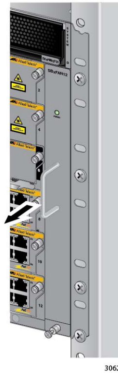
Figure 169. Loosening the AT-SBxFAN12 Fan Module from the Backplane Connector
