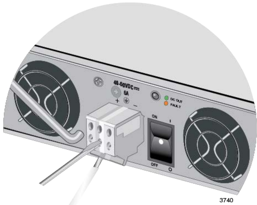
Figure 56. Connecting the Ground Wire to the DC Terminal Block
