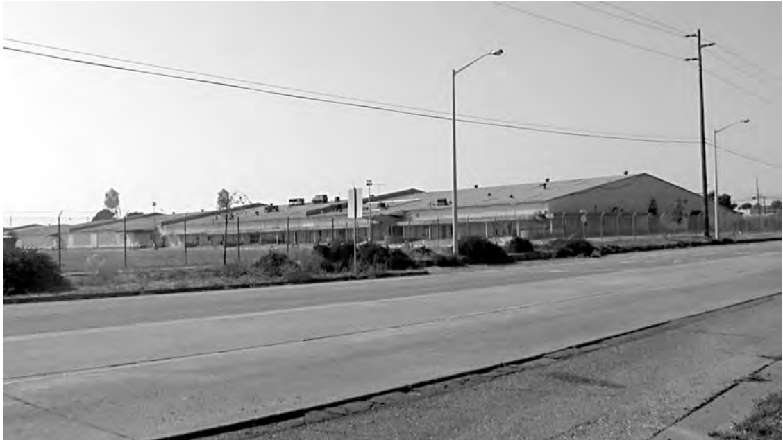
Figure IV.C-7 Views into Alameda Point from Main Street.
