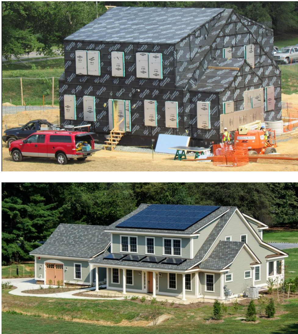
Figure 1. Construction of NZERTF showing the air barrier (top) and completed structure (bottom).
