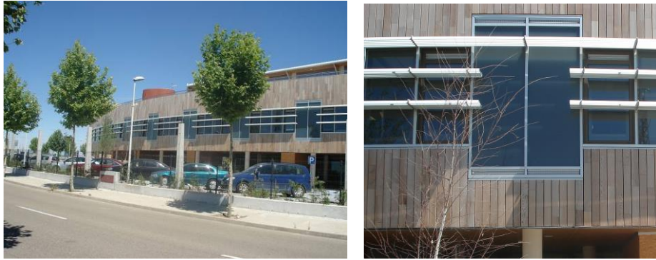
Figure 3: From left to right: view of the South façade of the building and detail of solar absorption chiller
