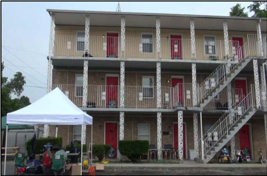
Figure 2: Simultaneously measurement of 9 apartments in multi-family residential building (NRCERT, 2011)
