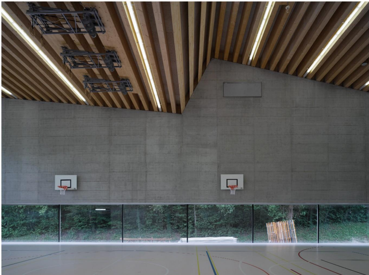
Figure 3. The design trick, to respect the architect wish for pure glazed openings was to dissociate air path from light path. On the picture we may see an opaque opening on the top of the space, guaranteeing evacuation of hot air on the top of the space and avoiding the creation of a hot buffer in the roof triangle. Glazing on the bottom offers only light and view.
