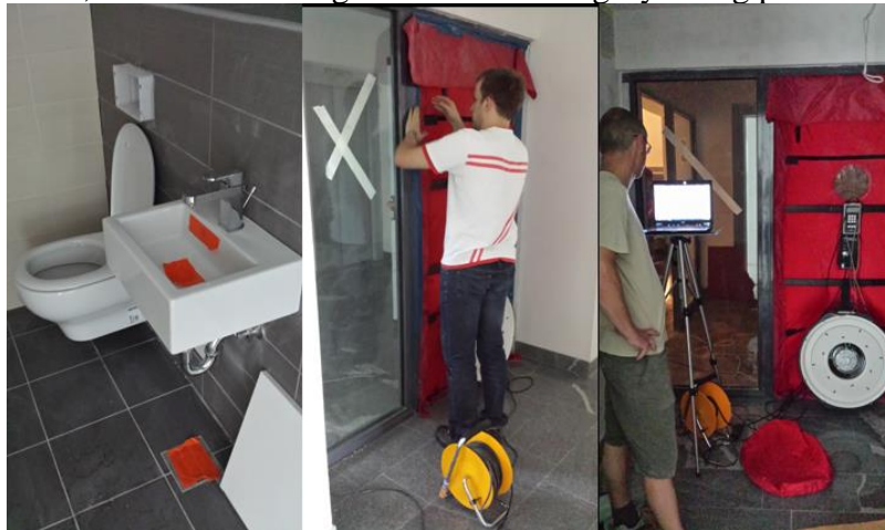
Figure 6: Preparation and execution of Blower door tests.
