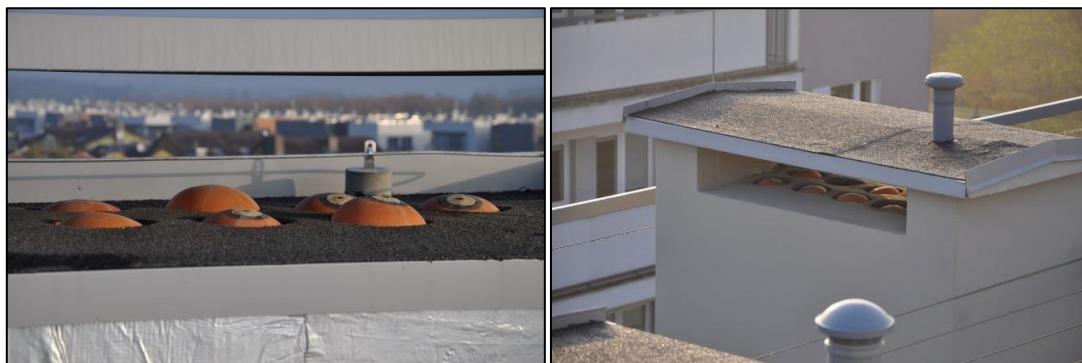
Figure 7: Extract ducts closed with use of inflatable inner rubber bladder
