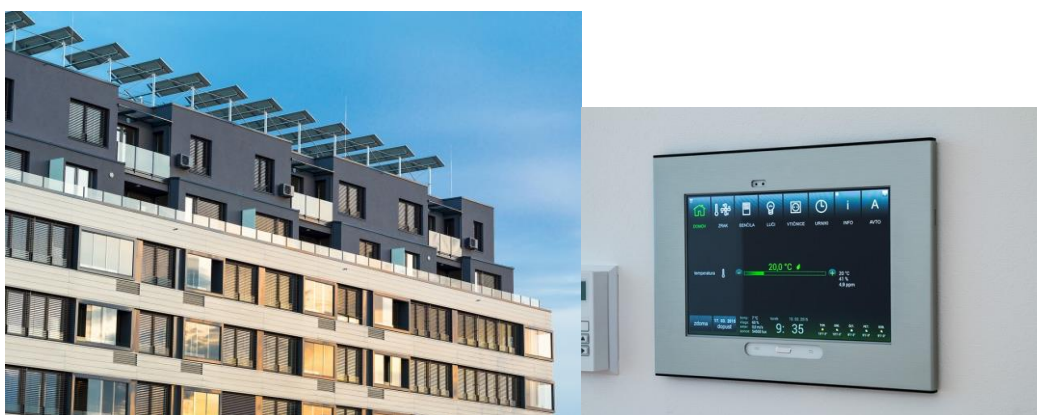
Figure 2: Eco-Silver House – PV power plant on the flat roof and the intelligent control unit in each apartment (Photo: Borut Slabe).
