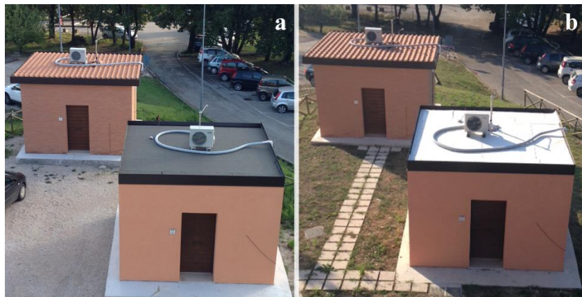
Figure 1: Continuously monitored buildings representing the field case study of the research.
