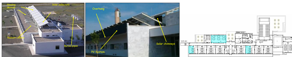
Figure 1. Different views of the building under study, showing schematically the different bioclimatic strategies implemented. To the right, a floor plan with the fully monitored offices in blue.
