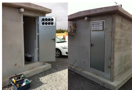
figure 1 Exhaust fans installed at the door of the test cell
