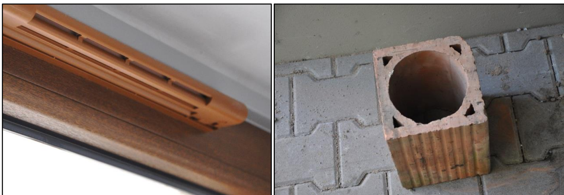
Figure 4: Trickle vents (left) and ceramic blocks used for extract ducts (right)
