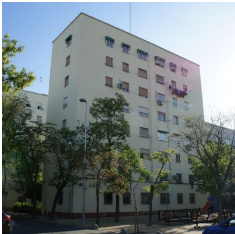
Figure 1: south façade of the demo case
