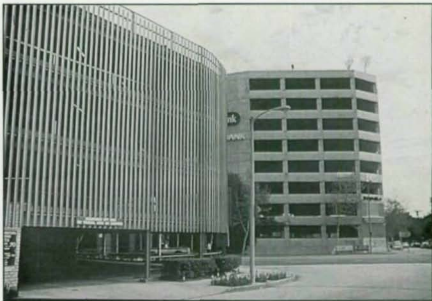
While a concrete garage in the Sherman Oaks area was substantially damaged by the Northridge Earthquake and needed to be closed, an older steel garage immediately across the street remained open. Photo courtesy of EQE Engineering.
