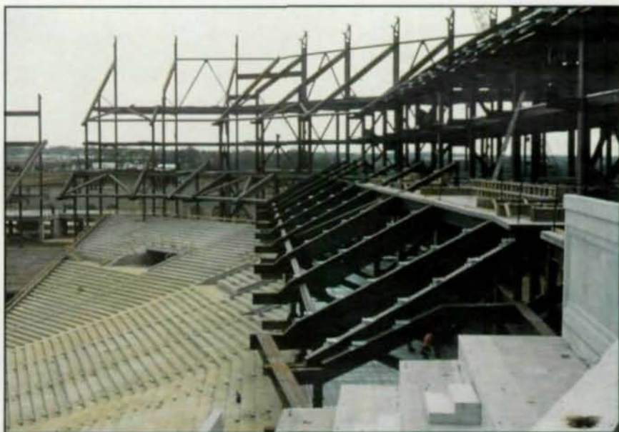
Shown above is the structural frame, looking down the firstbase side from the loge seating. The series of details at left show, from top to bottom: the connection of the precast seating to the steel; a close-up photograph of the connection; and a loge seating cross section.
