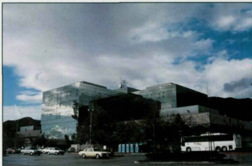
After the Olive View Medical Center collapsed during the Sylmar Earthquake in 1971 (top), it was rebuilt in steel (shown above after the Northridge Earthquake). Photos courtesy of EQE Engineering.
