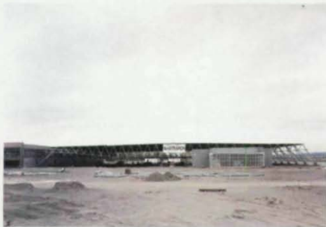
The 320'-wide hangar begins as a flat truss of nearly 400'...
