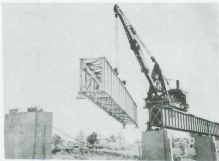
Figure 3 Grass River Bridge Girders
