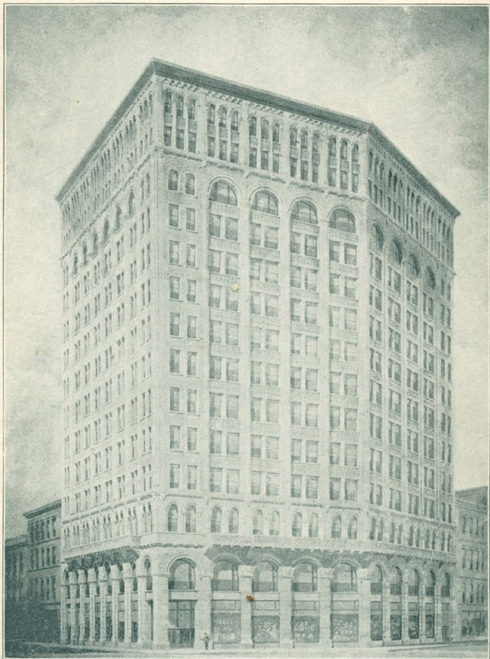
THE MABLEY BUILDING, Detroit. D. H. BURNHAM & CO., Architects. Godfrey & Hyde, Contractors. Steel designed by E. C. Shankland, Steel furnished by Schultz Bridge & Iron Co.
