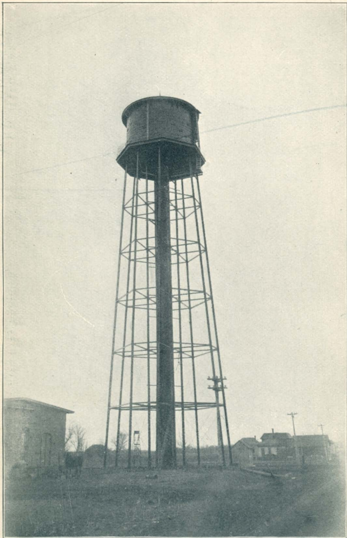
120 ft. WATER TOWER.
