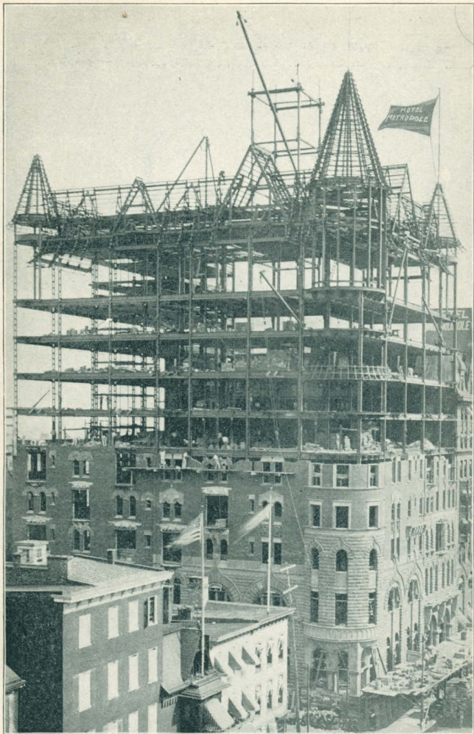
HOTEL WALTON, Philadelphia. Pencovd Iron Works, Contractors.
