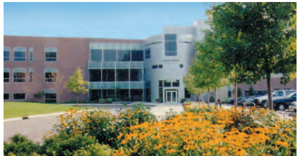
Parker Hannifin Corporation Headquarters Cleveland, Ohio
