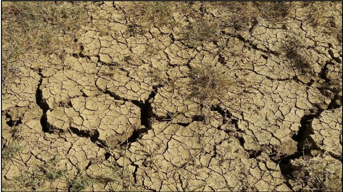
Figure 7.8 - Soil Structure within the Project Site (Shrinkage cracks)
