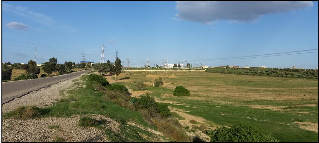
Figure 2.6 - STEG Electrical Substation
