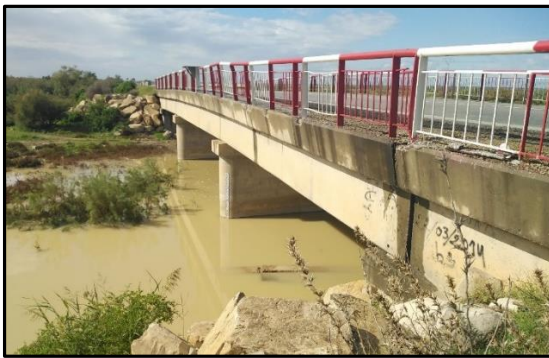
Bridge over Wadi Boughal
