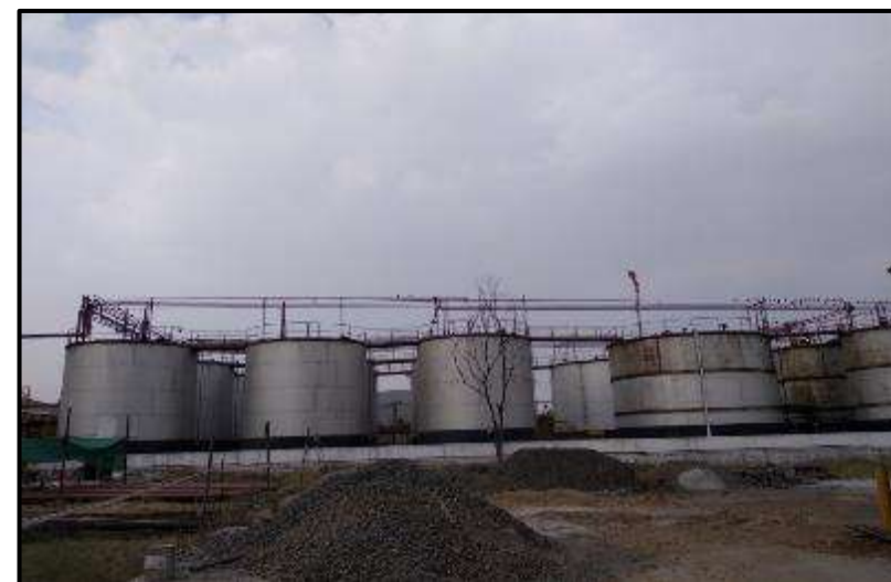
View: Oil Storage Tank
