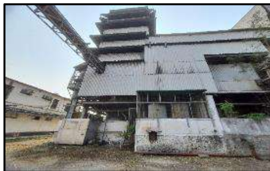
View: Palm Refinery Source: GAA
