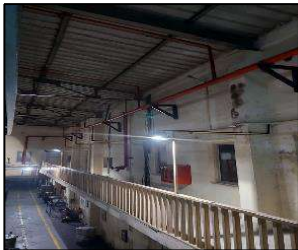
View: 1 st floor corridor
