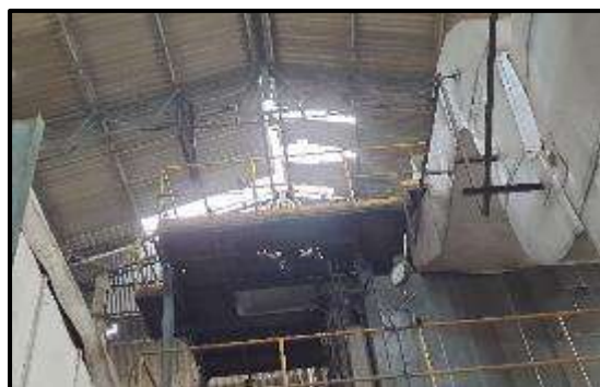
View: Bulk flow conveyor Source: GAA
