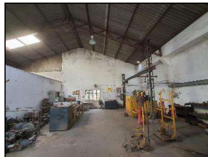
View: Technical Room
