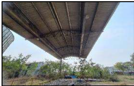
View: Loading Unloading Source: GAA
