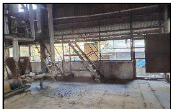
View: Refinery Source: GAA
