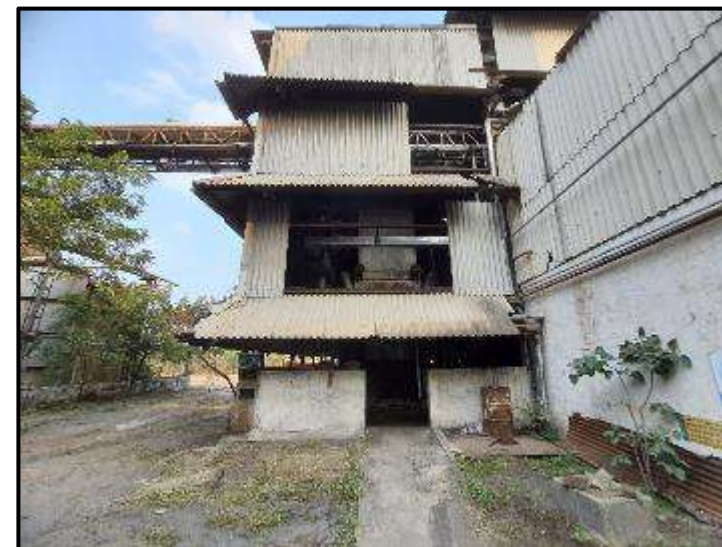
View: 12 TPH Boiler House
