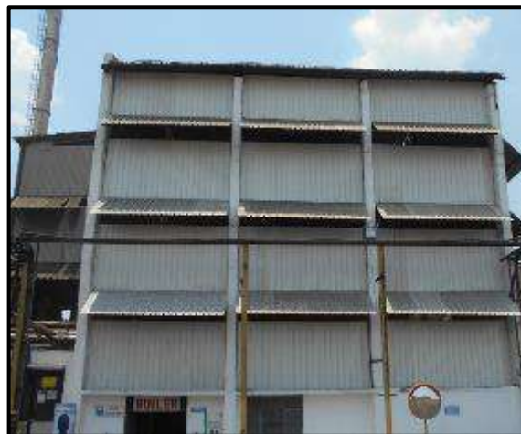
View: Boiler House
