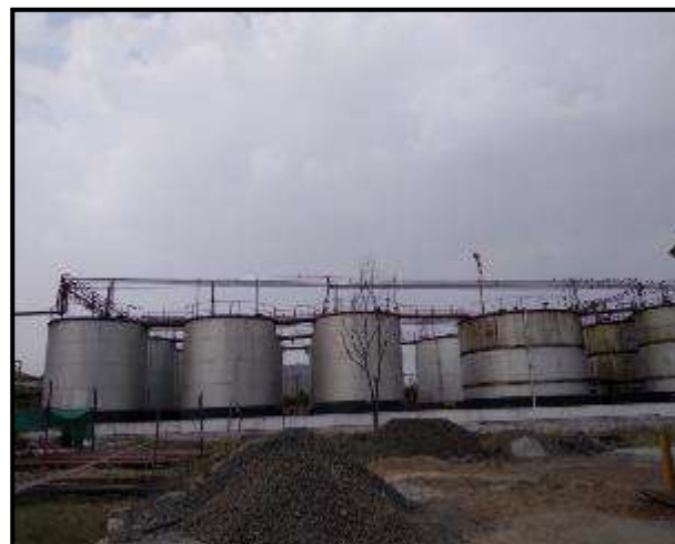
View: Oil Storage tank
