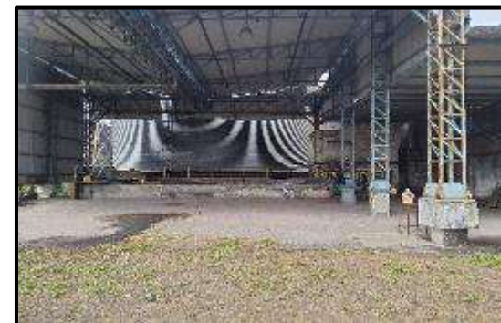
View: Silo Shed Source: GAA
