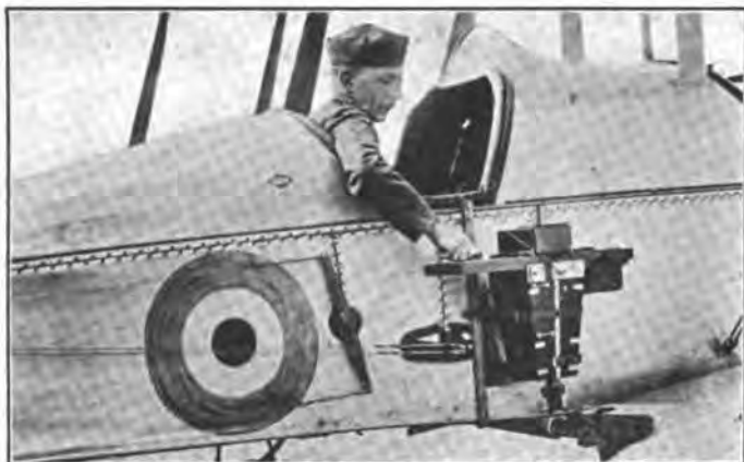
THE MOUNTING OF THE CAMERA ON BRITISH OBSERVATION PLANES
