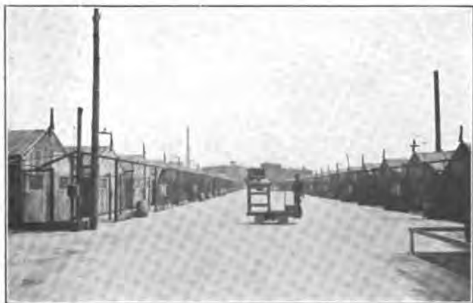
OUTDOOR TEST SHED AT THE LIBERTY MOTOR PLANT OF THE NORDYKE AND MARMON COMPANY, APRIL, 1918
