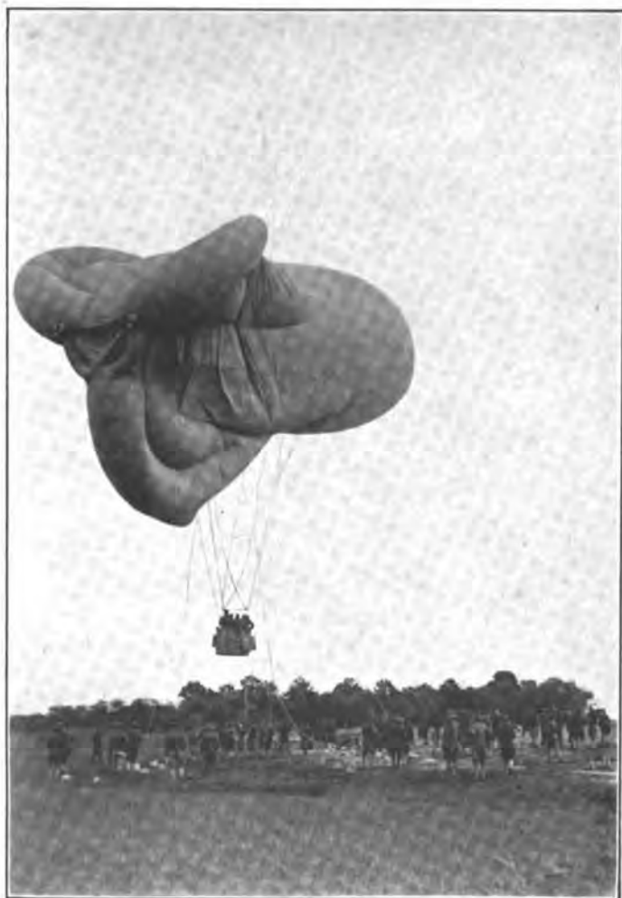
THE CAQUOT BALLOON ASCENDING; THE TRIPLE-LOOPED TAIL IS INFLATED BY THE WIND, AND NOT ONLY KEEPS THE HEAD TOWARD THE WIND, BUT BY MEANS OF A DIAPHRAGM ARRANGEMENT INSIDE THE BALLOON KEEPS THE MAIN GAS BAG RIGID EVEN WHEN MUCH OF THE HYDROGEN HAS LEAKED OUT
