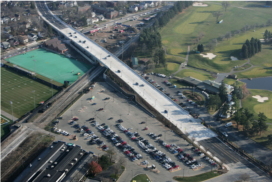
Stadium Bridge Replacement
