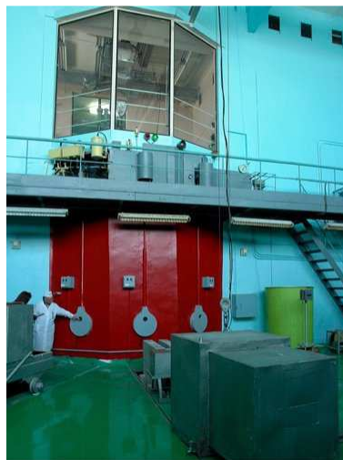
FIG. 4. Ground view of IR-100 reactor.
