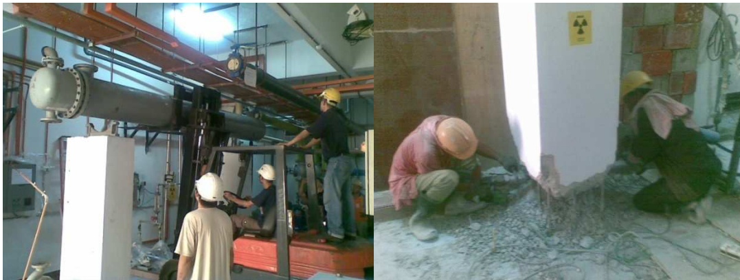
FIG. 3. Dismantling shell and tube heat exchanger.
