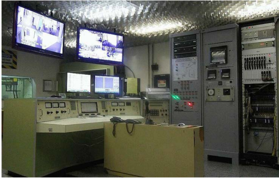
FIG. 5. Reactor control room with control console for the data acquisition system and closed circuit television surveillance.
