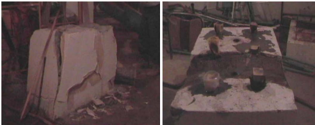
FIG. 2. Concrete pedestal demolition with the use of expansive chemicals.
