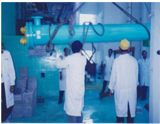
FIG. 3. Handling of heat exchanger [5].
