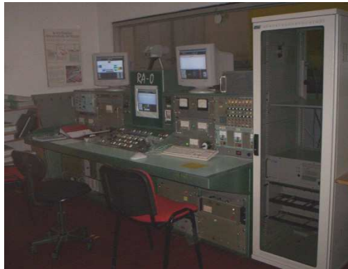
FIG. 2. Control console view.
