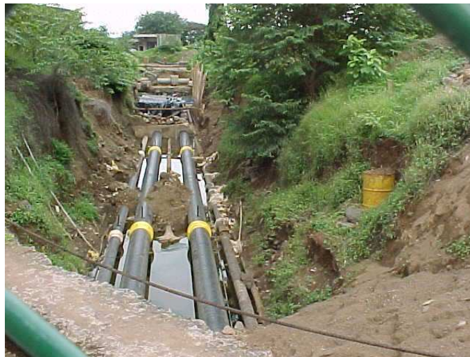
FIG. 6. Repaired subsoil primary coolant piping.
