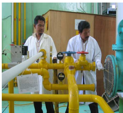
FIG. 7. Heat exchanger tubes inspection conducted in 2006 [6].
