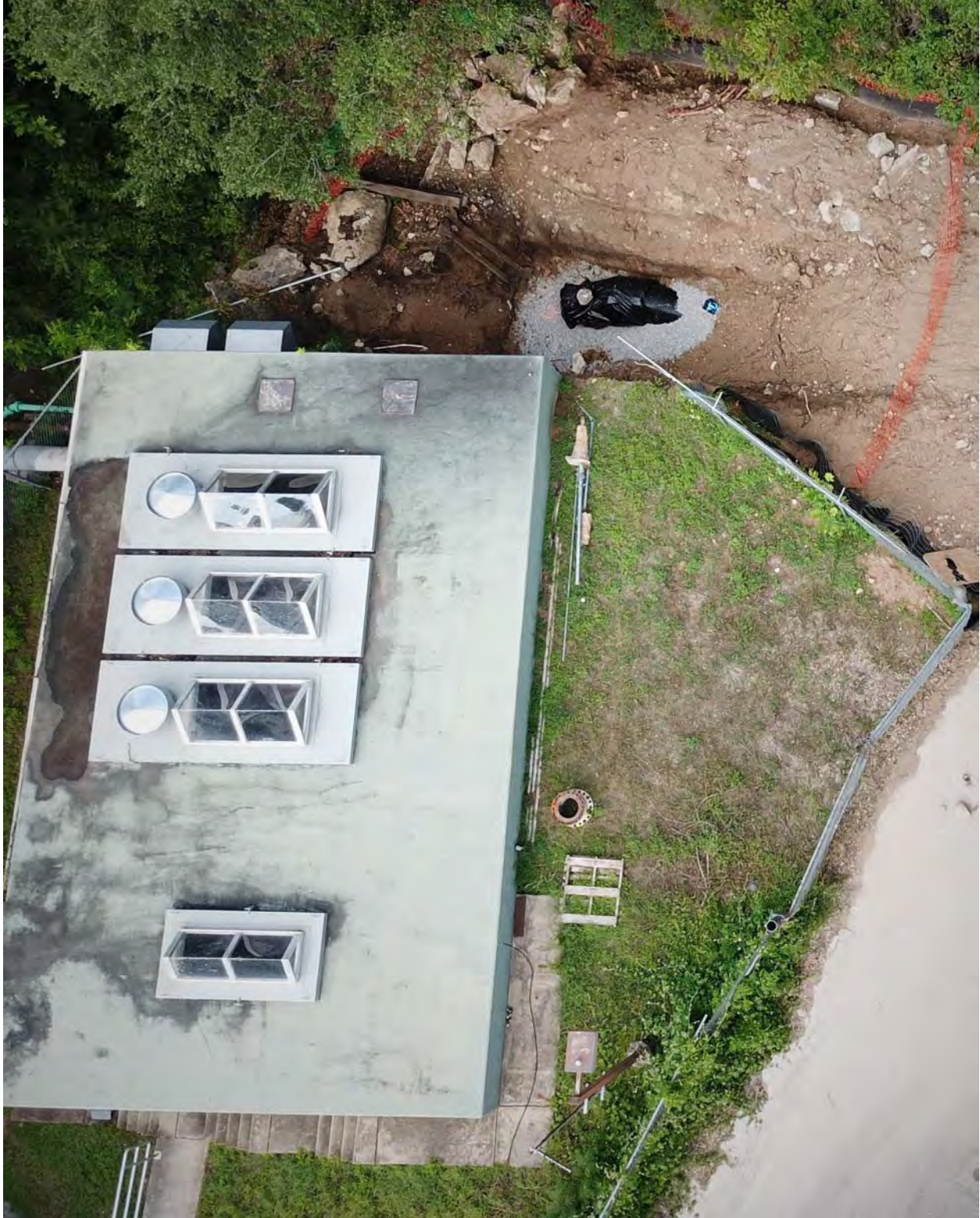
RWL 2 Pump Station Tie-In
