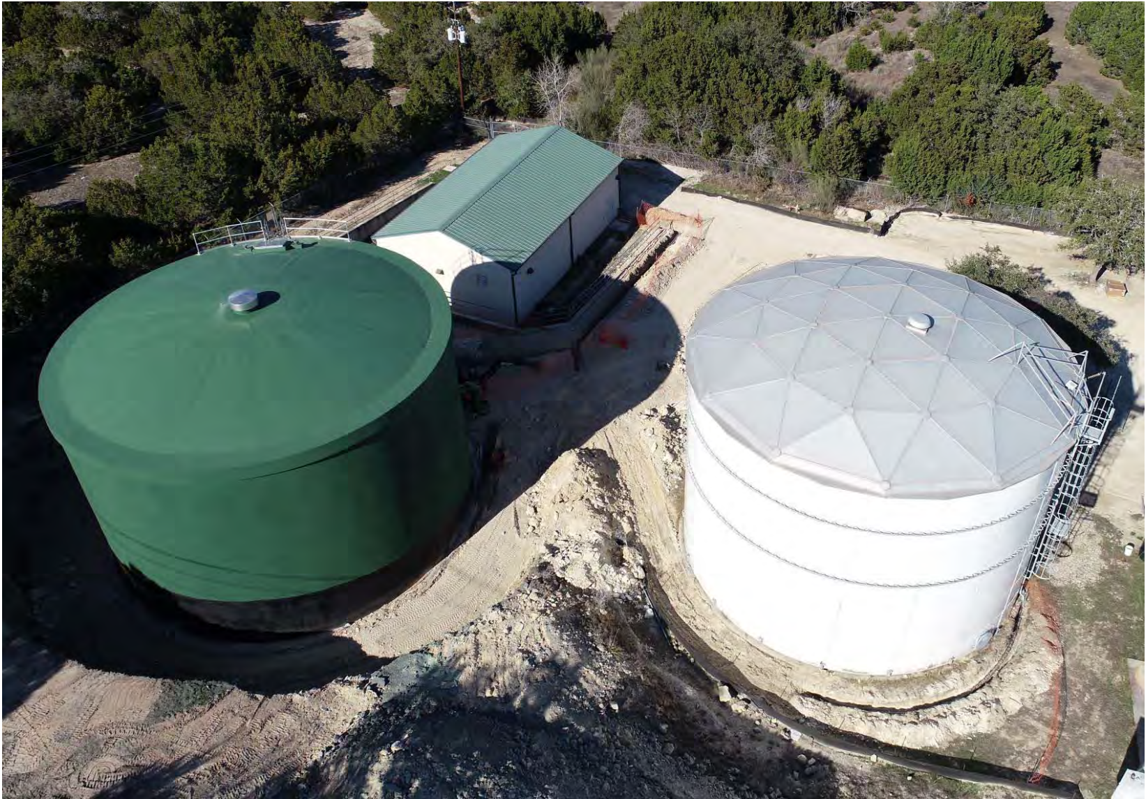
Bee Cave Pump Station GST 2 Site
