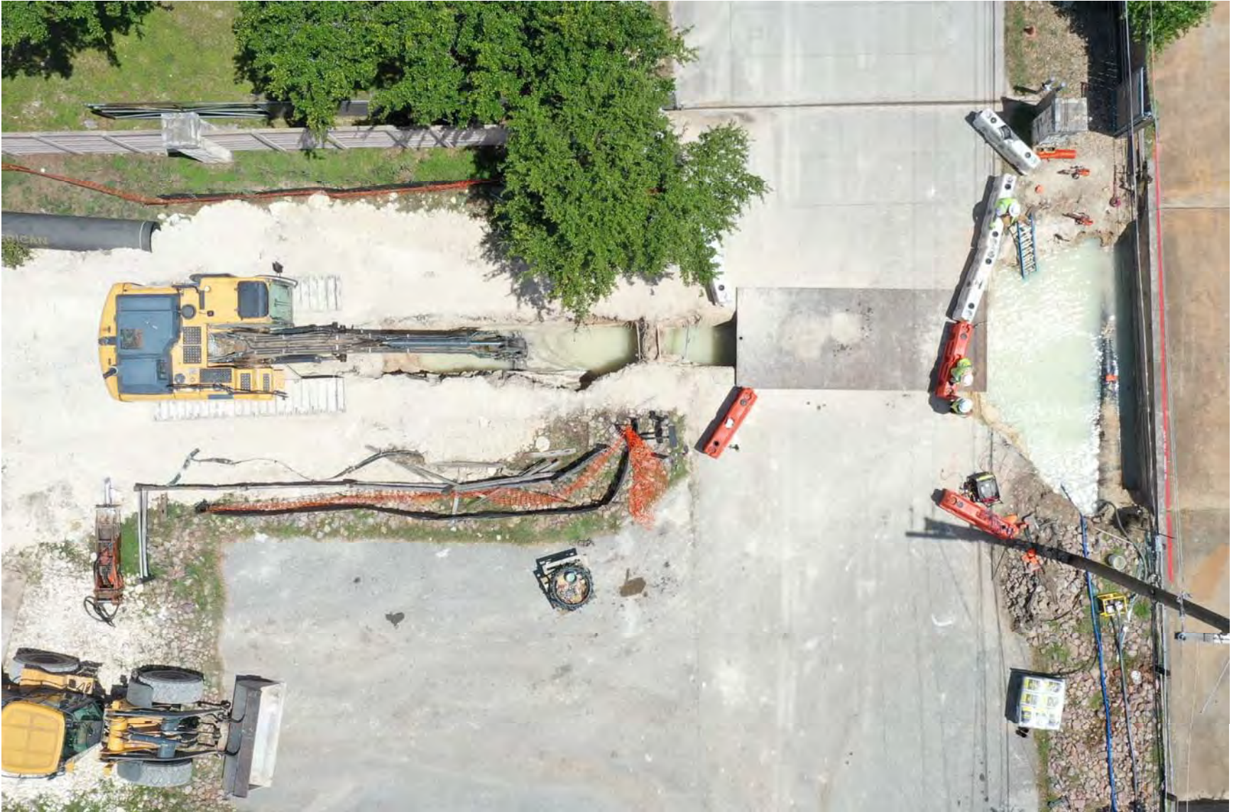
RWL 2 Tie In at Uplands WTP
