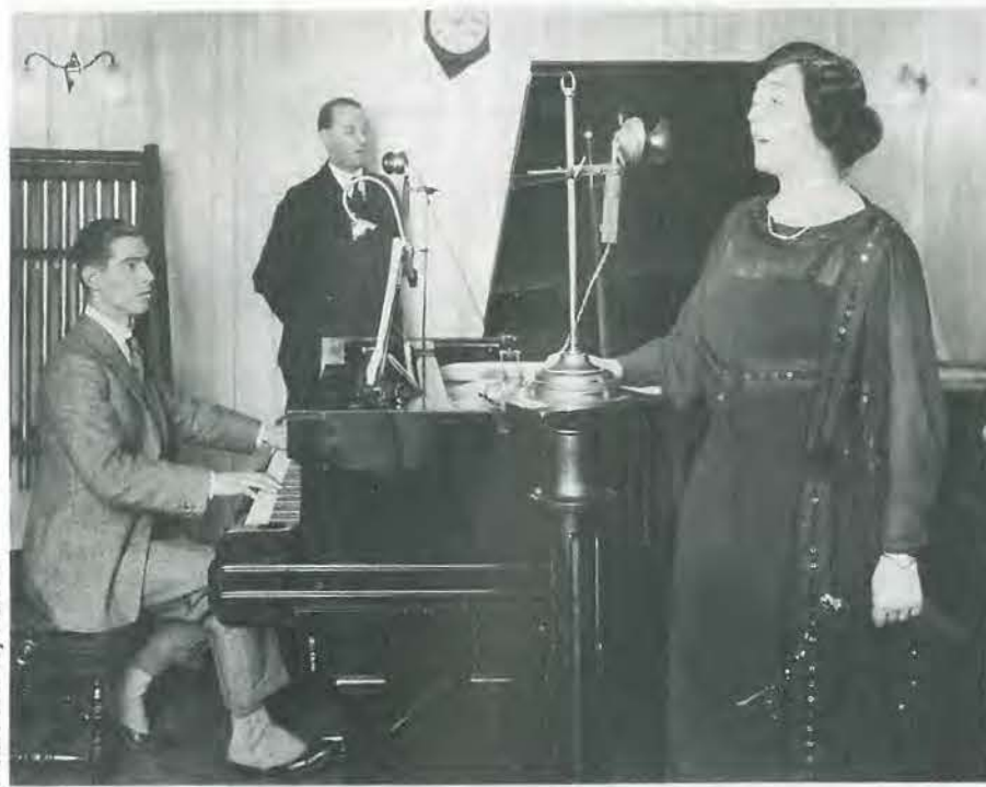
Music recital in 1922 from the 2LO broadcasting studio in London. Miss Olive Sturgess sings into a carbon-granule telephony hand microphone fixed in a laboratory-style clamp, raised to the required height on a decorative pot stand. Also singing is Mr John Huntingdon, while the accompanist in spats is Mr R Stanton Jefferies.
