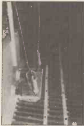
From left: British flag – plywood lead-in-trunk for minimum shunt capacitance – brass bells shield lead through insulators from spray and rain, but they are shunted by unprotected strain insulators; Italian flag – steel mesh offers neither protection from weather nor reduction in shunt capacitance; British flag – no trunk at all – cheaper and quicker to cut holes in wall, but efficiency of shielding bells on horizontal insulators is doubtful – bells shunted by unprotected strain insulators (seems to be universal practice).
