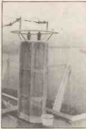
From left: British flag – plywood lead-in-trunk for minimum shunt capacitance – brass bells shield lead through insulators from spray and rain, but they are shunted by unprotected strain insulators; Italian flag – steel mesh offers neither protection from weather nor reduction in shunt capacitance; British flag – no trunk at all – cheaper and quicker to cut holes in wall, but efficiency of shielding bells on horizontal insulators is doubtful – bells shunted by unprotected strain insulators (seems to be universal practice).
