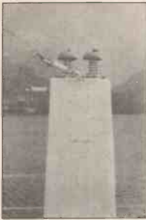
From left: British flag – plywood lead-in-trunk for minimum shunt capacitance – brass bells shield lead through insulators from spray and rain, but they are shunted by unprotected strain insulators; Italian flag – steel mesh offers neither protection from weather nor reduction in shunt capacitance; British flag – no trunk at all – cheaper and quicker to cut holes in wall, but efficiency of shielding bells on horizontal insulators is doubtful – bells shunted by unprotected strain insulators (seems to be universal practice).
