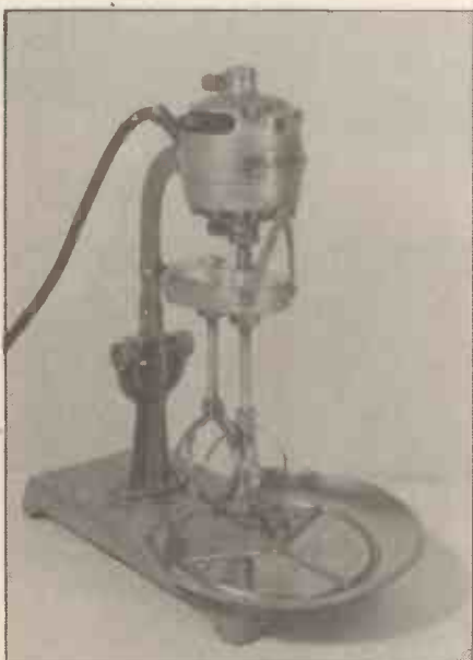
Getting back to the basics: an early electric eggbeater, c. 1920; with no handle and precious little insulation, it was definitely not intended for portable use!
