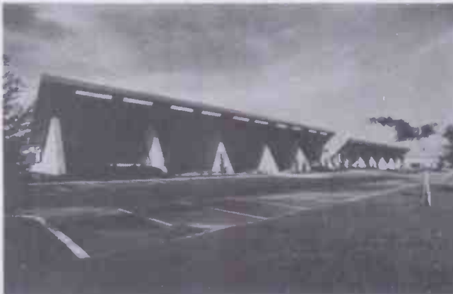
Above. The sloping roof of the factory acts as a solar collector.
