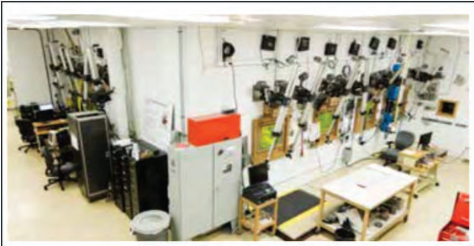
Figure 9: Outside a Westinghouse Commercial plant high-level cell.
