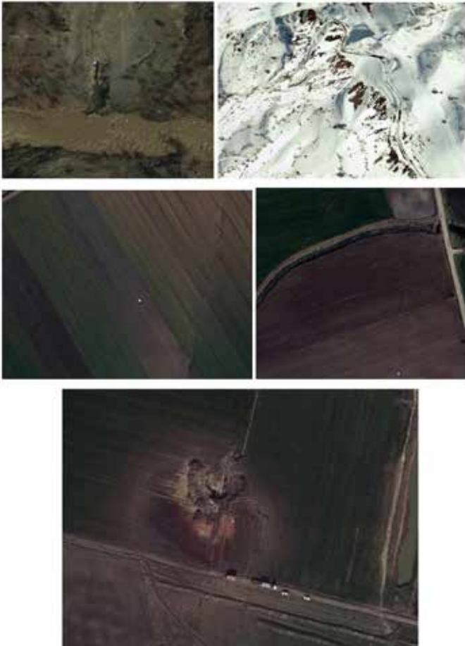
Fig. 1: Aerial images from the natural gas pipeline damages sourced from landslides, fault flowering, liquefaction and lateral spread. Aerial image credit: HGM Küre platform of General Directorate of Mapping, Türkiye.
