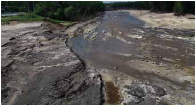
Fig. 1: Failed Edenville Dam.
