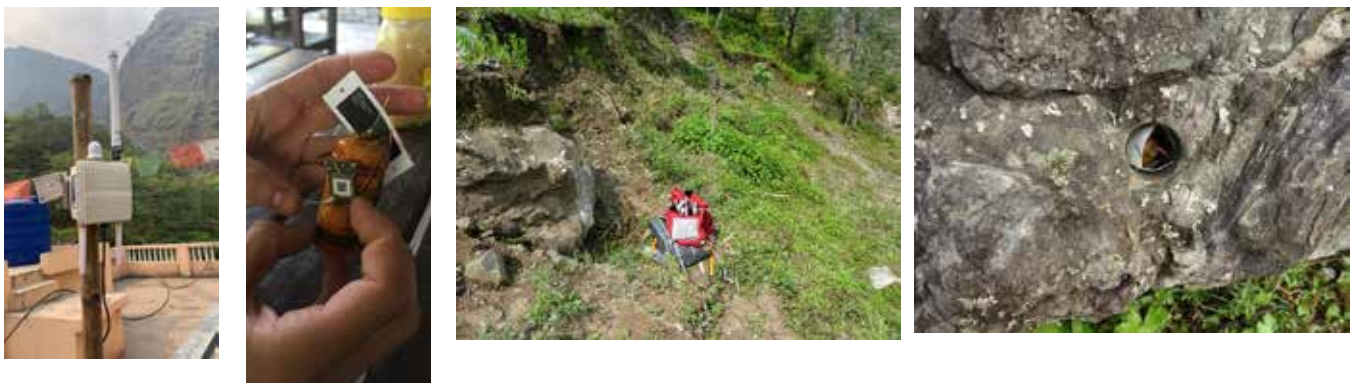
Fig. 3: (a) Gateway installed at the location of Fig. 2 (b) Boulder tag/tracker (c) example of boulder in landscape selected for monitoring landslide (d) Installed tag in boulder.
