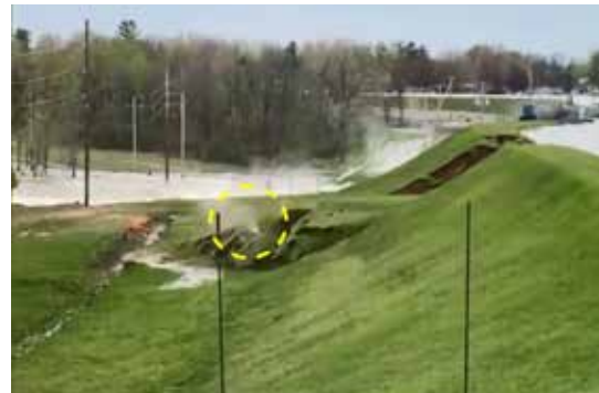
Fig. 2: Water jets emanating from slide mass during failure.
