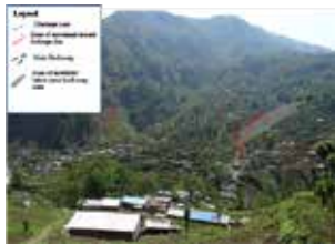
Fig. 2: View from gateway looking towards landslide and drainage lines monitored with tags
