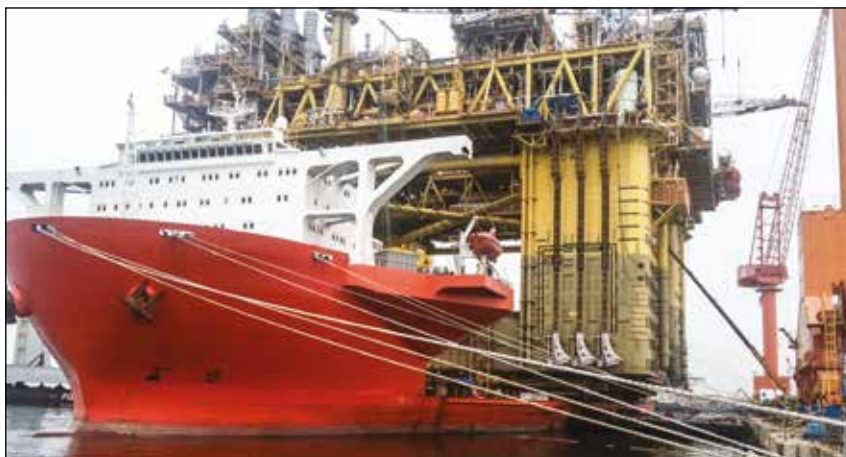
▲ The superlifting and launch of a 43.000-ton floating oil production system in Malaysia for the Gumusut-Kakap offshore field has set high benchmarks for safety through its use of sophisticated EVO-Series synchronous hydraulics to lift, balance, weigh and smoothly launch massive resource structures.
