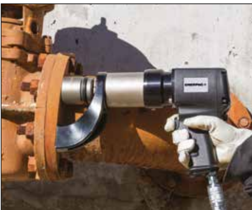
◀ The PTW1000 makes quick work of this flange maintenance job.
