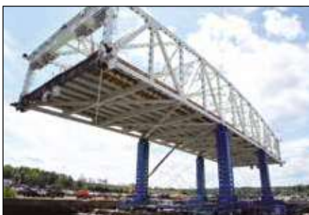
Incremental bridge lifting
