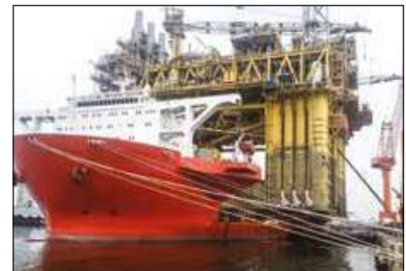
Synchronous superlift and launch
