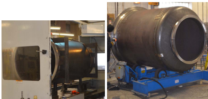
Figure 3: The two sections of the large volume vacuum can under construction at Meyer Tools.
