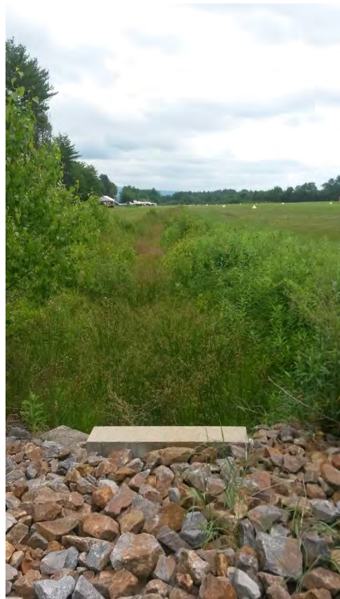
Wet Ditch on North Side of Runway
