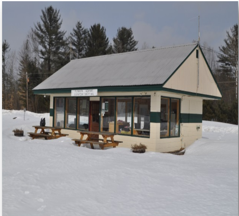
Figure 2.10. Airport Administration Building Photo by Stantec (February 2014)
