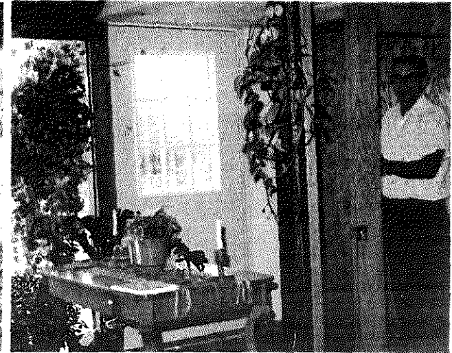
INNOVATIVE ENTRY - Harold Ling shows glass door which pulls out from wall to form air lock entry when wood panels are inserted behind table. This kept living room of earth shelter free from wintry blasts. (Nancy Pouler Photo)
