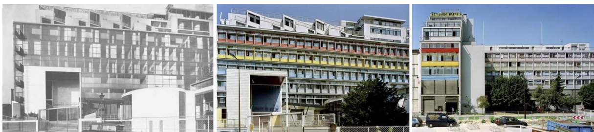
Figure 4. Cité de Refuge, Paris: outdoor of the building over time [22-23].
