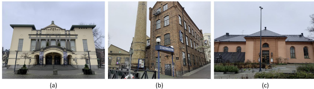
Figure 1. Three historic buildings are selected for case studies. (a) Östgötateatern, (b) Stadsmuseum, and (c) Hörsalen.
