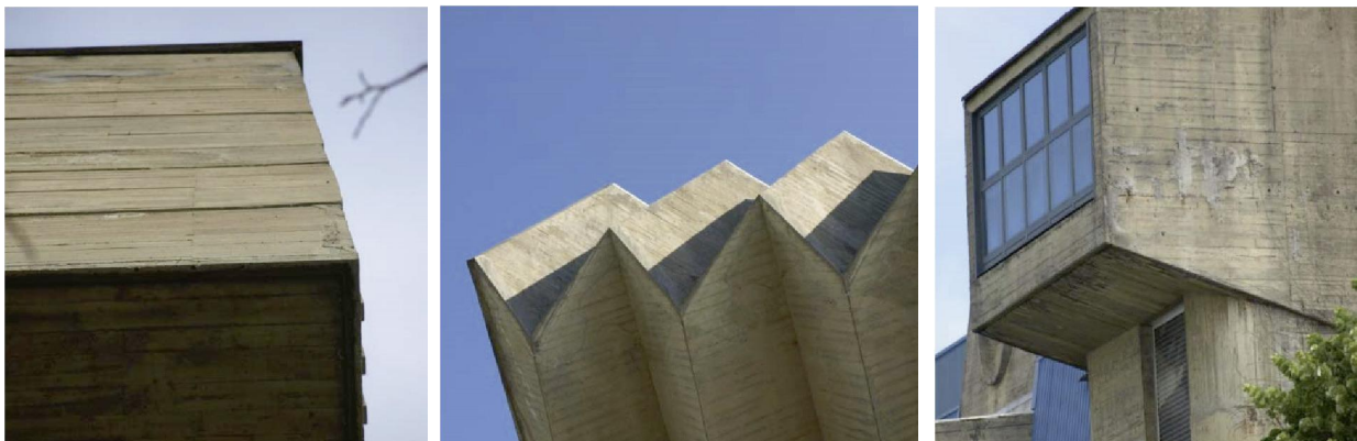
Figure 2. Detail of concrete of the three buildings.
