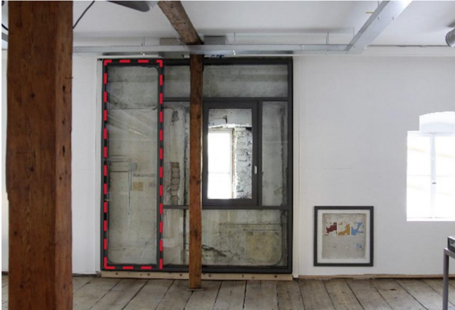
Figure 1. Transparent internal wall insulation on the west-side in the upper floor of the Alte Schöfferei. The left part of the transparent internal wall insulation (dashed rectangle) is examined and evaluated.
