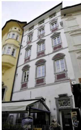
Figure 1 Reference building of Climate zone I (Portici house-I), Piazza Erbe 11, Bolzano
