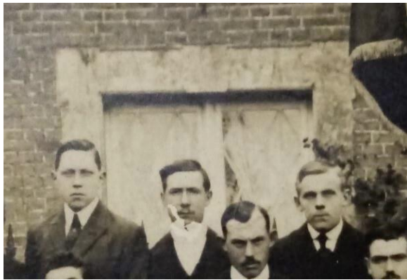
Figure 2: Original appearance of the windows
