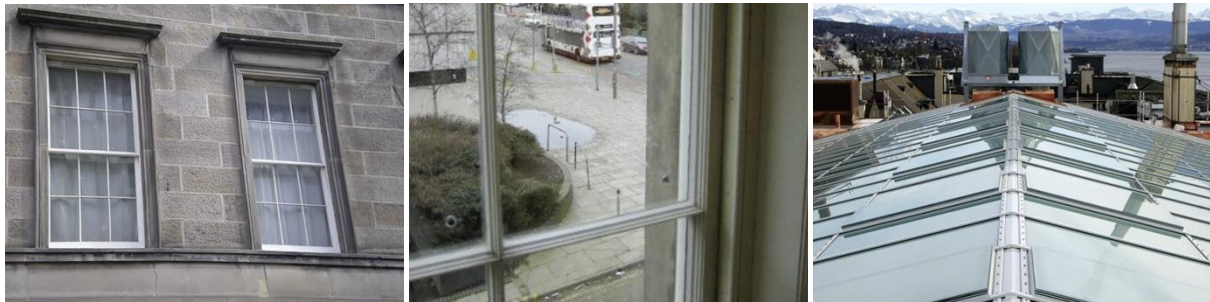
Figure 3 (a, b). Vacuum glazing installed in a historic building located in Edinburgh. Source: [17]
