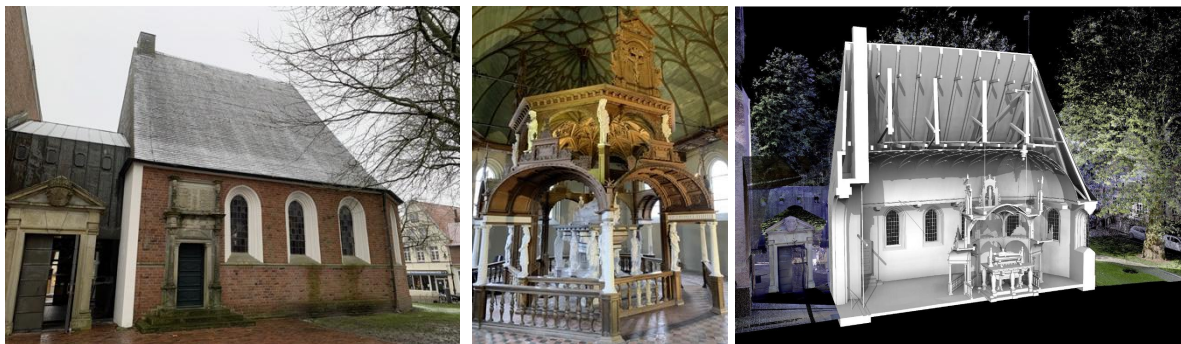
Figure 1. Exterior view (left), interior view (middle) and the point cloud based 3D-model (right) of the Edo-Wiemken-Monument in Jever (source 3D-model: DhochN-Nord Digital Engineering GmbH).
