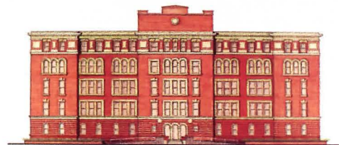
An 1898 New York City public school will be revived as a 241-bed AIDS facility (above) by Perkins & Will/Davis, Brody & Associates.
