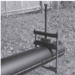
Figure 15 Mechanical Re-Rounding Clamp Installed
