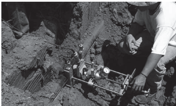
Figure 3 Saddle Fusion Repair
