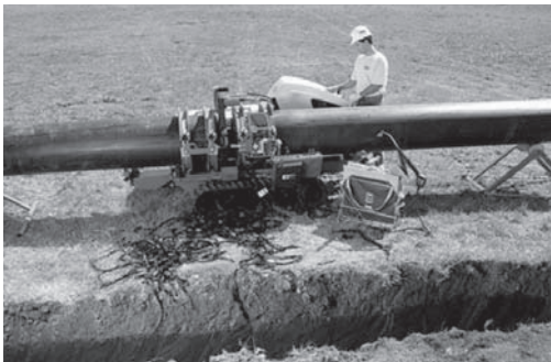
Figure 1 Above Ground Repair with Fusion Machine
