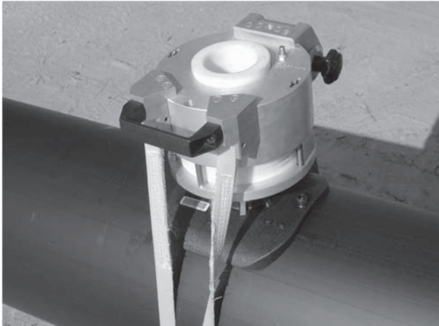
Figure 4 Electrofusion Patch Repair
