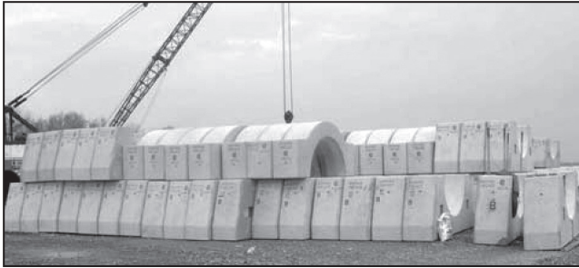
Figure 3 Two-piece Concrete Anchors in Storage at Marine Job-Site
