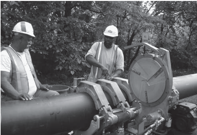
Figure 1 Joining Large Diameter PE Pipe with Butt Fusion
