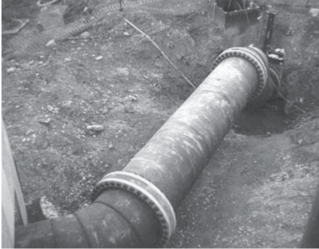
Figure 13 Flange Adapter Assembly
