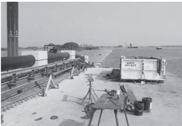
Figure 4 PE Pipe Weighted and Floated for Marine Installation
