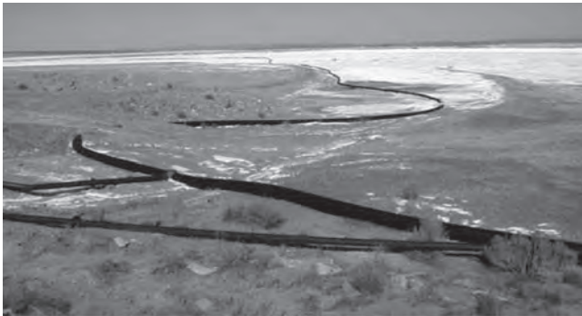
Figure 2a On-grade Installation of PE Pipe in an Industrial Application. Note "snaking" along right of way.
