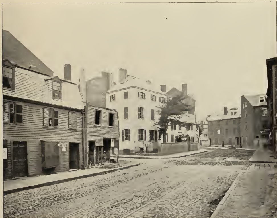
VI.f. — TREMONT STREET BEFORE WIDENING, 1869. Looking North from Pleasant Street
