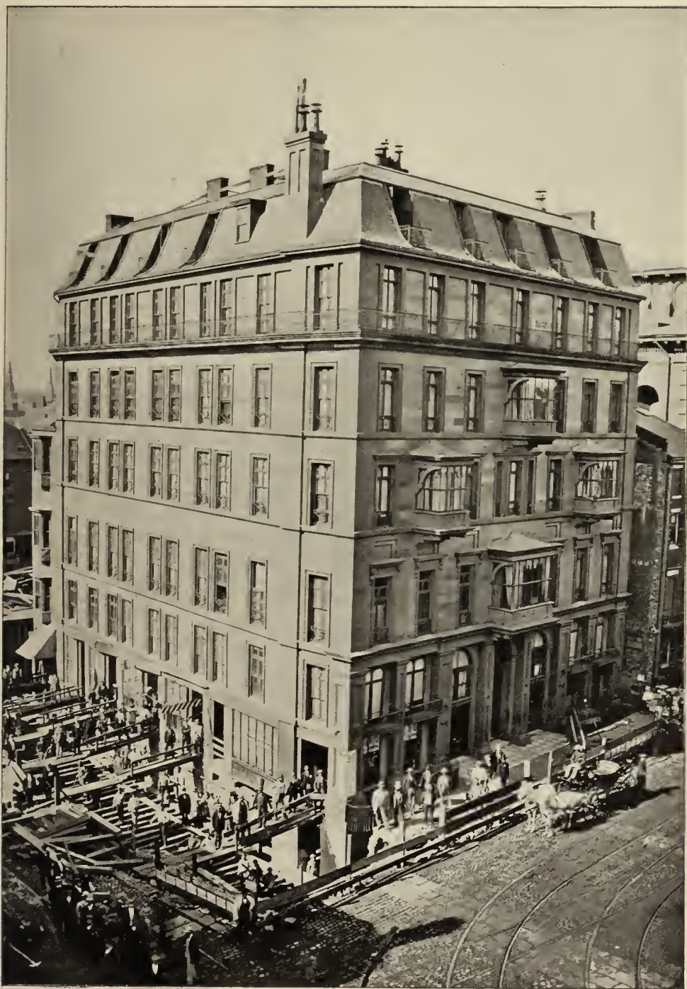
VII.a. — REMOVAL OF HOTEL PELHAM, 1869.
