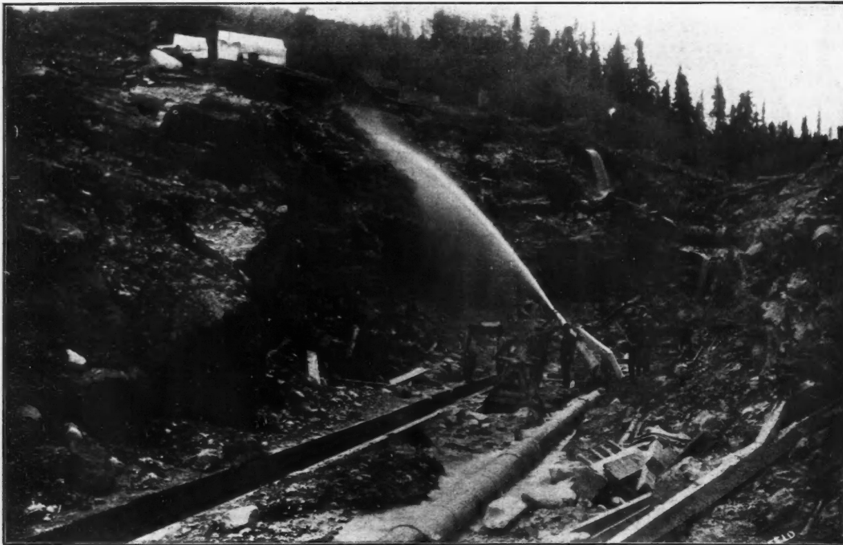
HYDRAULICKING BY DE LAMARE SYNDICATE, BOULDER CREEK, ATLIN, B. C.
