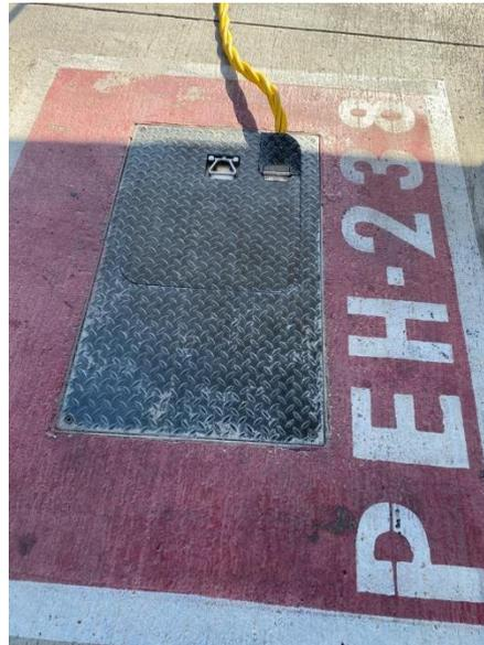
Figure 51 - Ground fixed GPU
