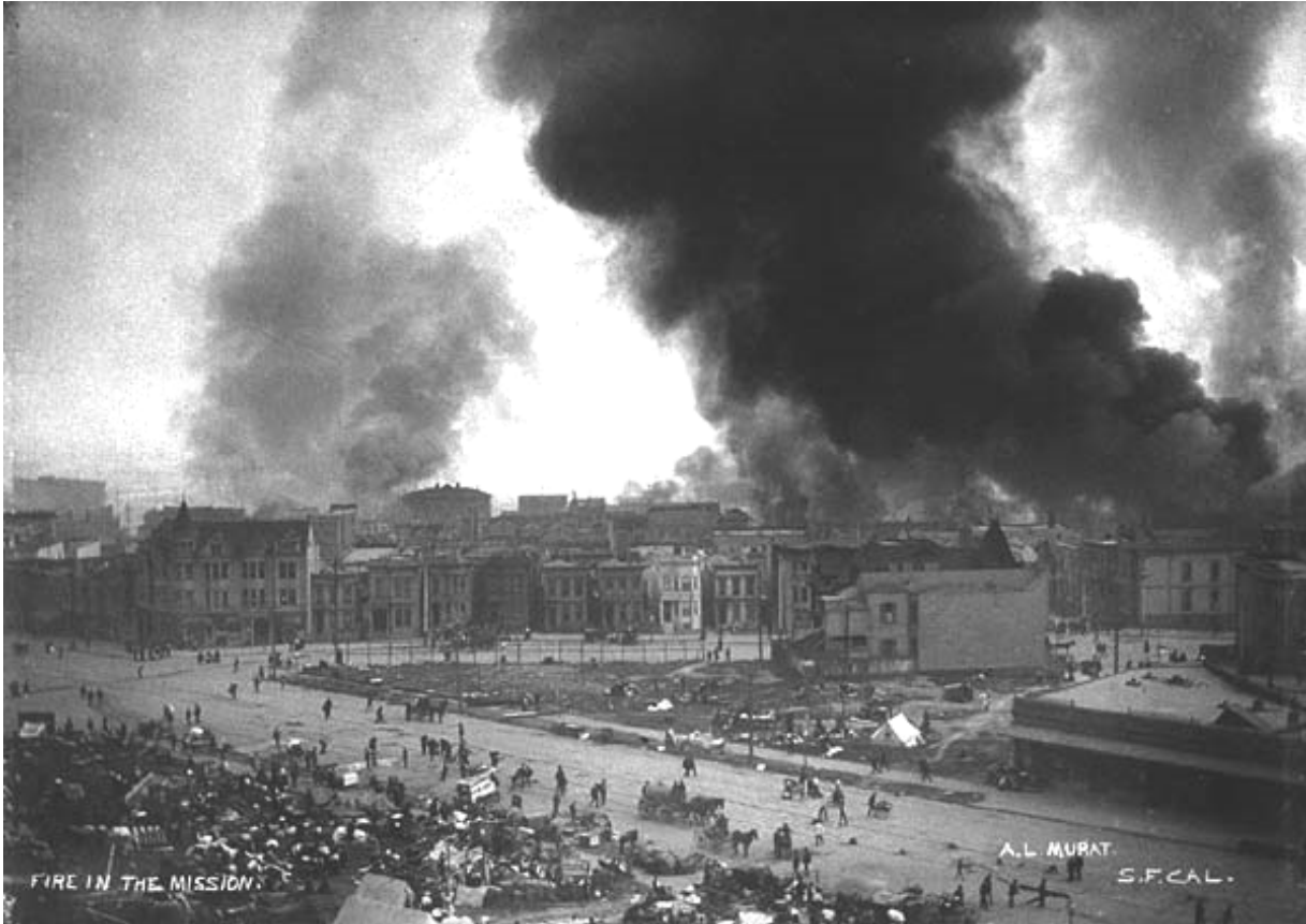
“View from Laguna and Market Streets of the Great Fire Burning through the Mission District.” Museum of the City of San Francisco. Web. http://www.sfmuseum.org .
