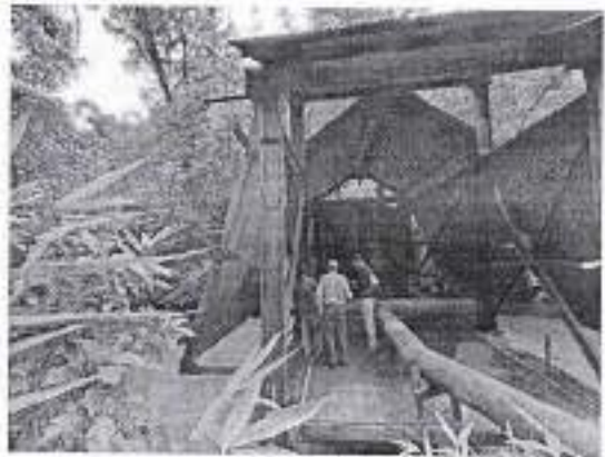
Fig:19 Pump house beside Lunar river
