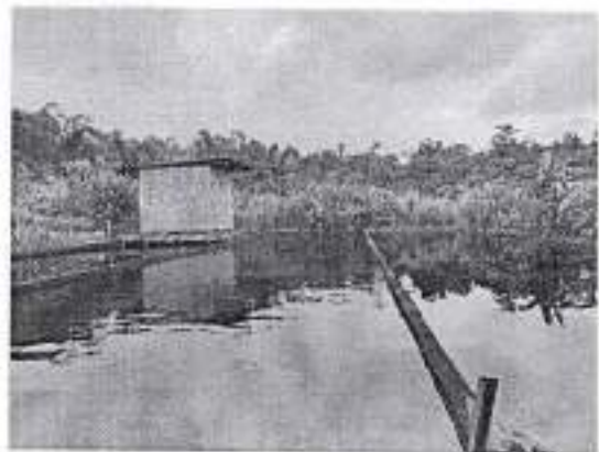
Fig:21 River water settling tank
