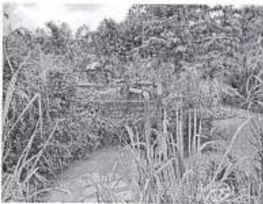
Fig:20 Pump house beside Umparthi river
