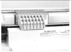
Fig. 15 Control circuit terminals
