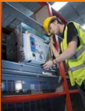
Direct Response Engineer Installing Retrofit ACB
