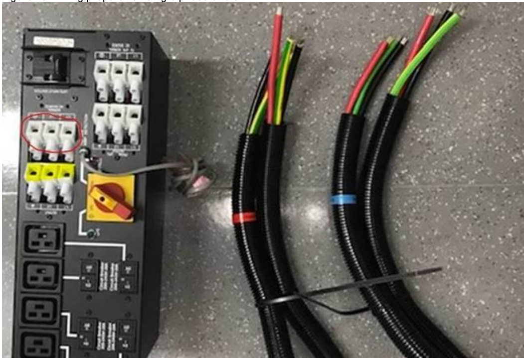
Figure 28: Wiring preparation single phase UPS unit
